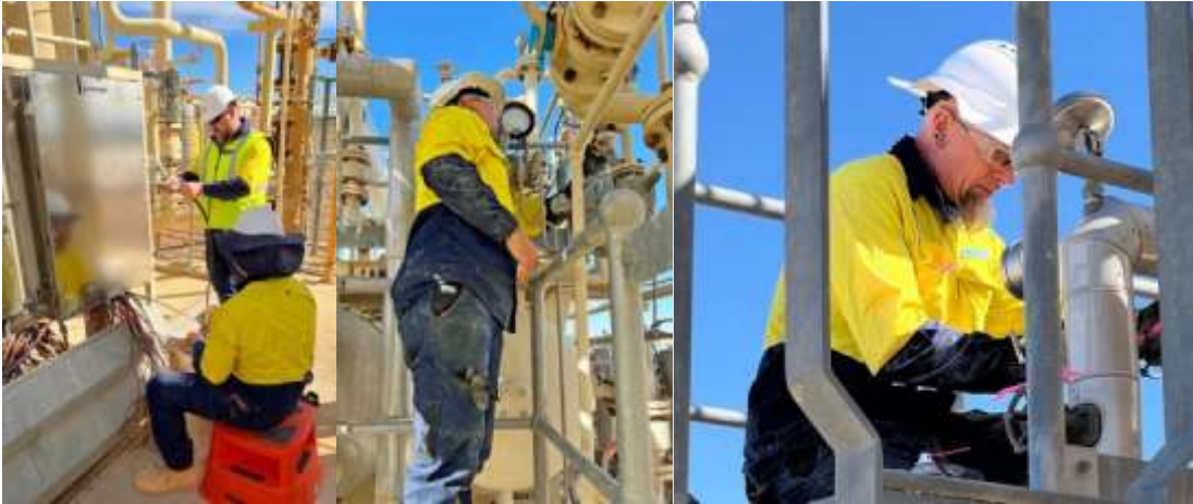
Refurbishment works underway at Eromanga
