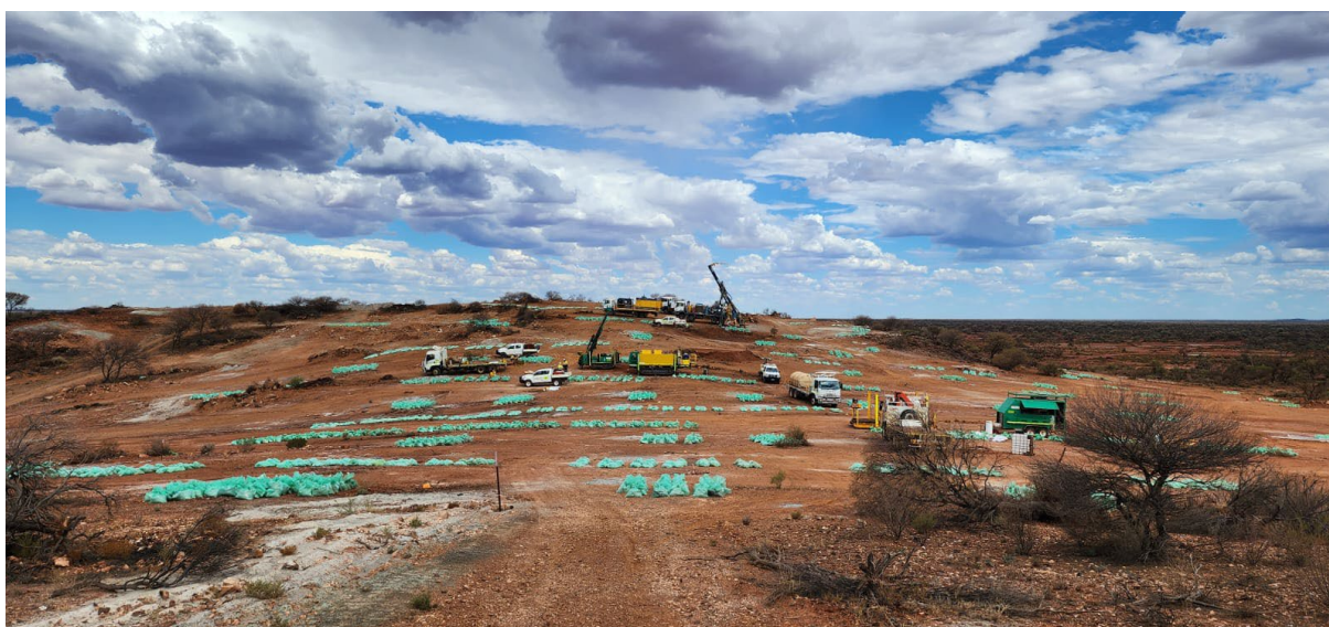
Plate 2 – RC grade control and geotechnical diamond drilling in progress at Saturn's planned Apollo Hill bulk sample pit location. Photo taken 21 February 2023.
