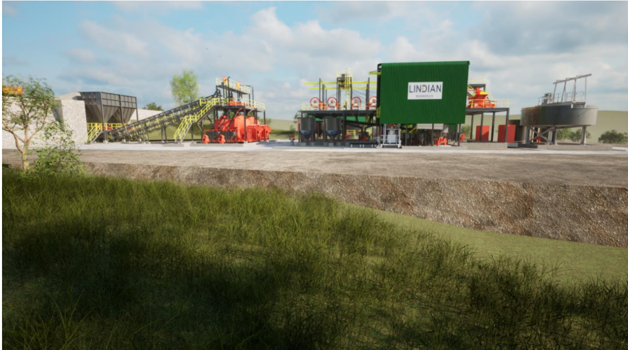
Image 7: Preliminary schematic of plant design from ground level. Existing retaining wall (left), ball mills (centre left), recovery circuit (centre) and tailings thickener (right)
