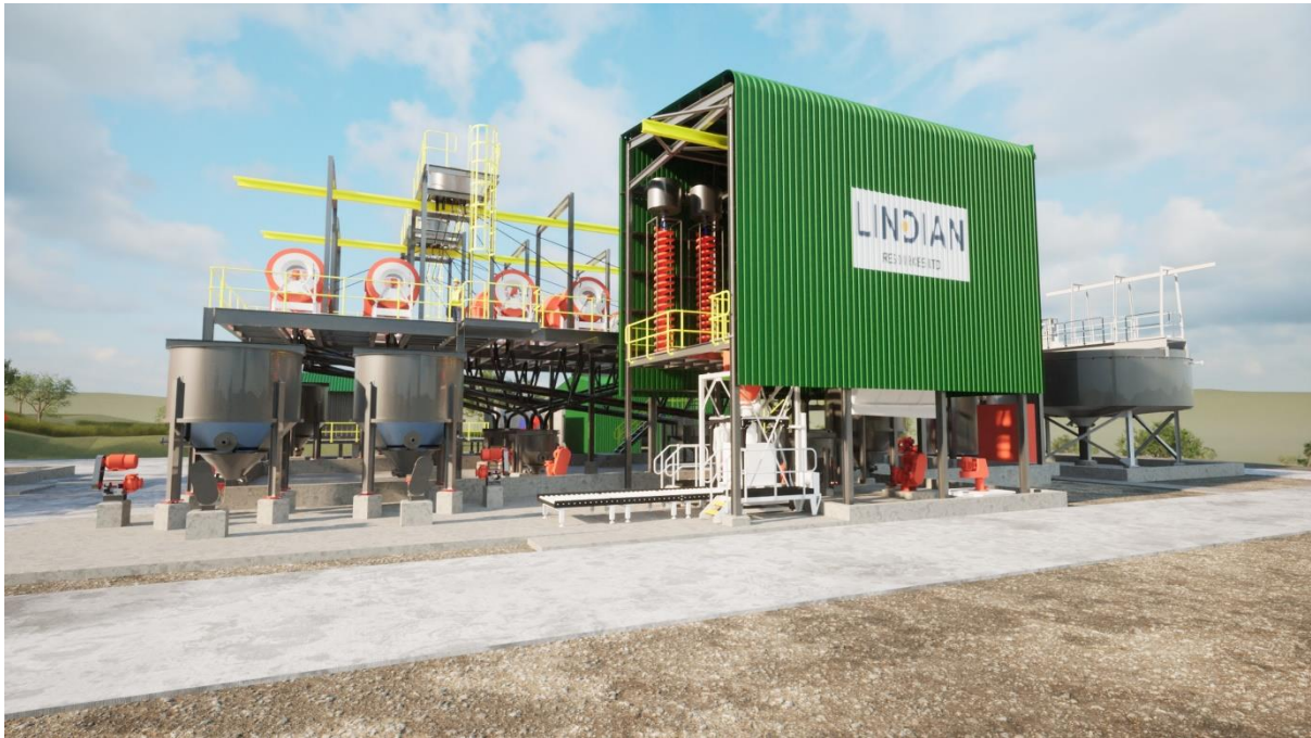
Image 10: Side view (artistic) of the recovery circuit and concentrate filter press and packing shed and tails thickener.
