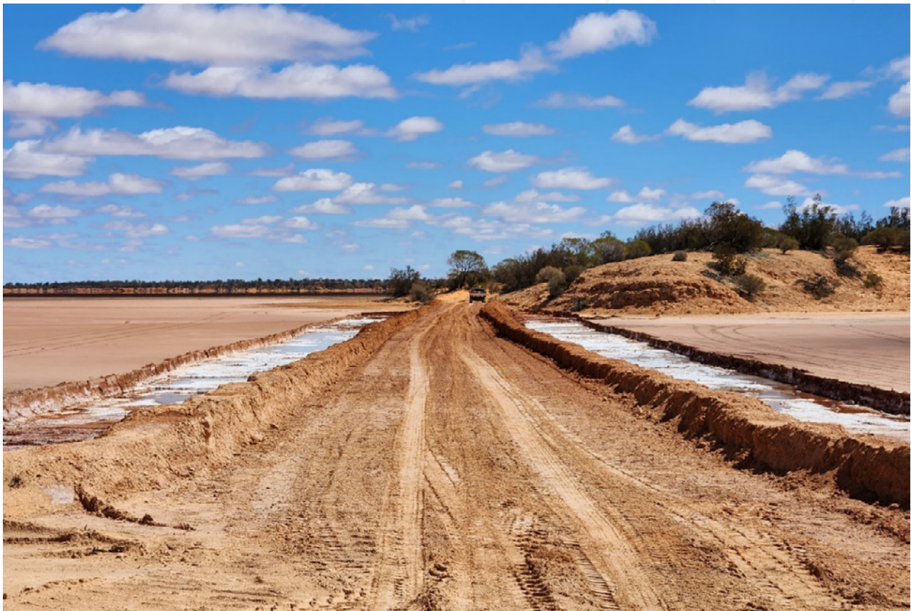
FIGURE 2: CAUSEWAY ACROSS LAKE SURFACE TO FACILITATE DRILLING CAMPAIGN
