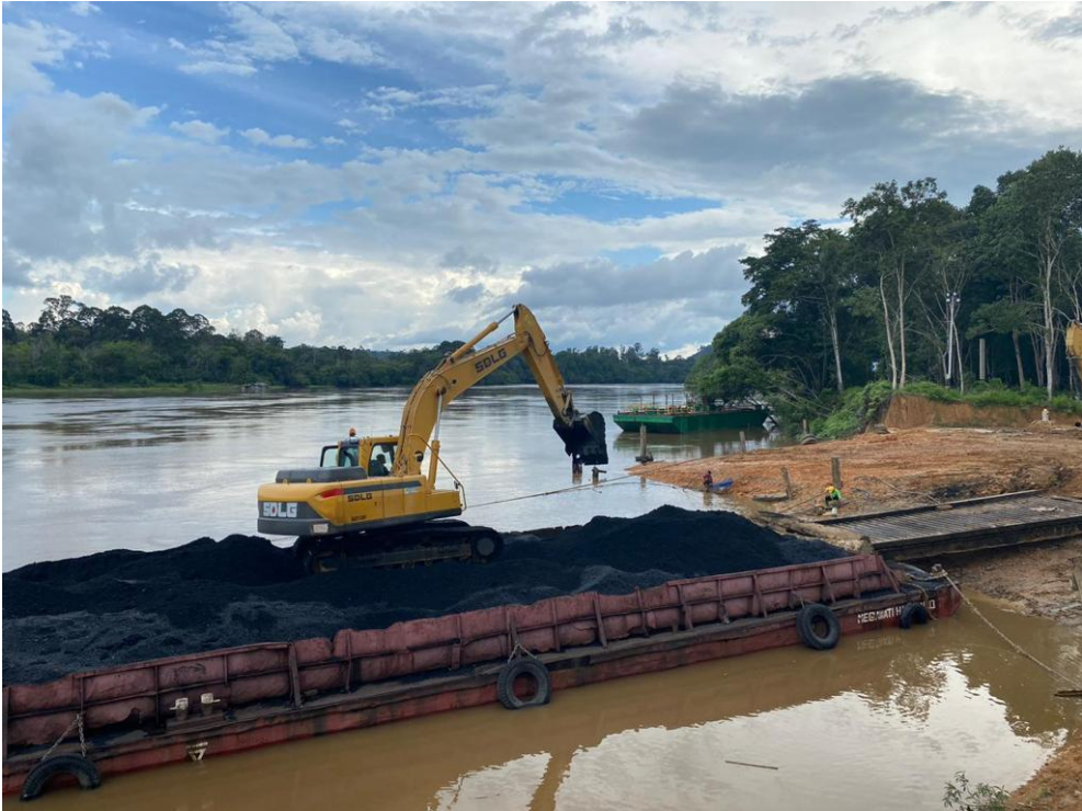
Coal loading onto barges at the Batu Tuhup Jetty
