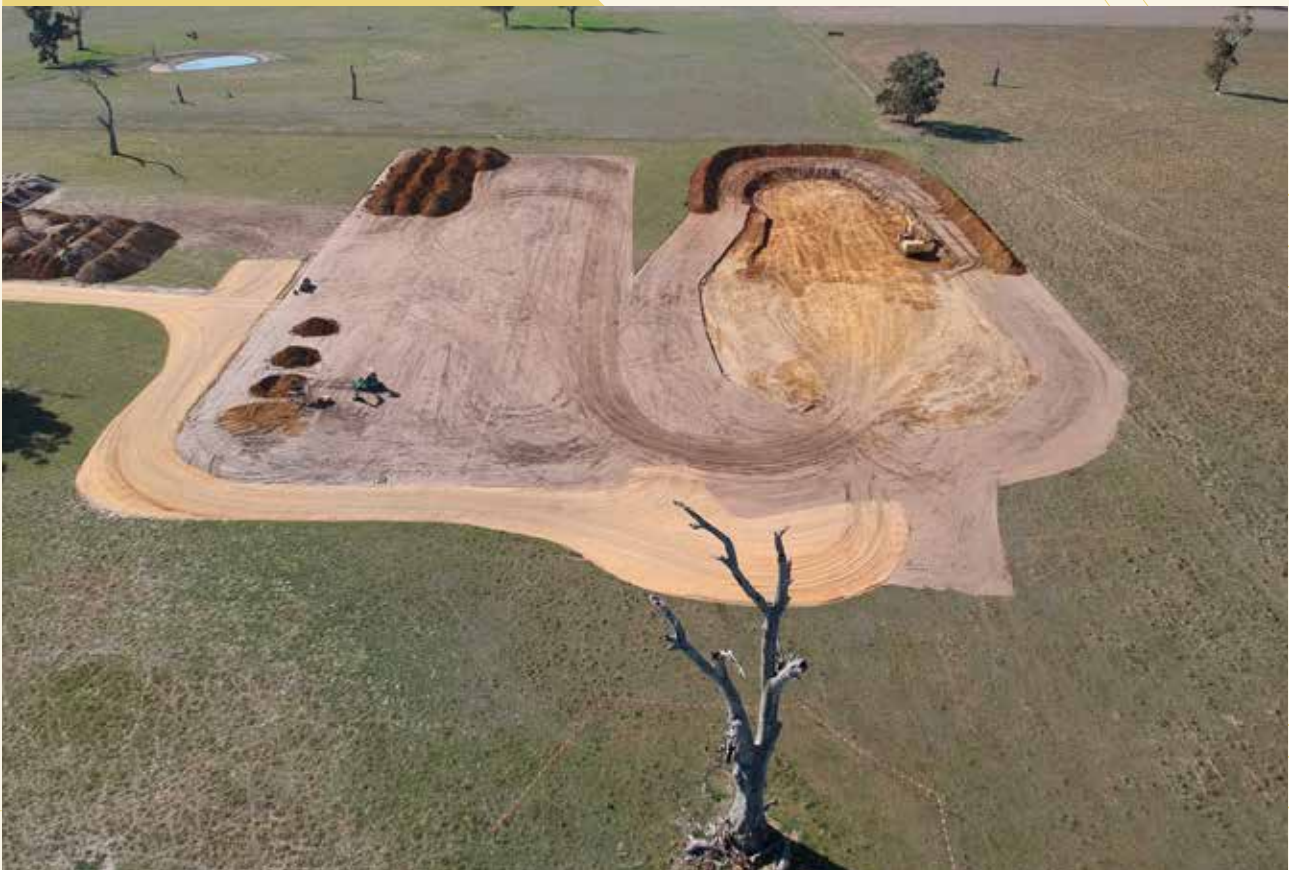
May 2022 - Aerial view of trial mining pit
