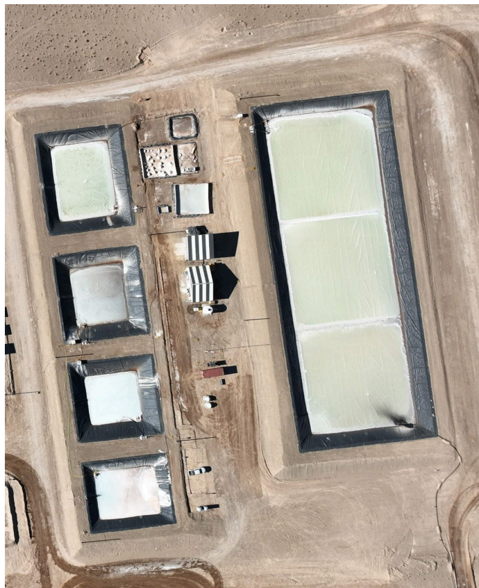
Figure 12: Aerial view of existing pilot plant
