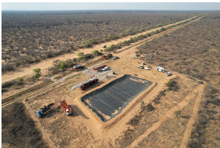
Figure 4 - Serowe-3.1 site in preparation for flow-testing.
