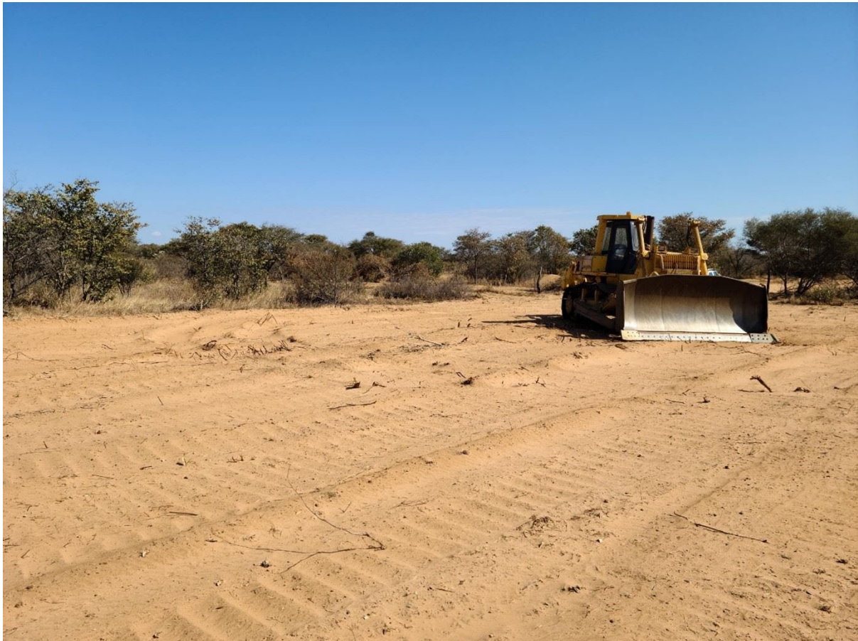
Figure 3 - Serowe 7 site cleared for drilling.
