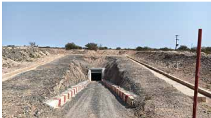
Figure 2: Portal access to the underground workings
