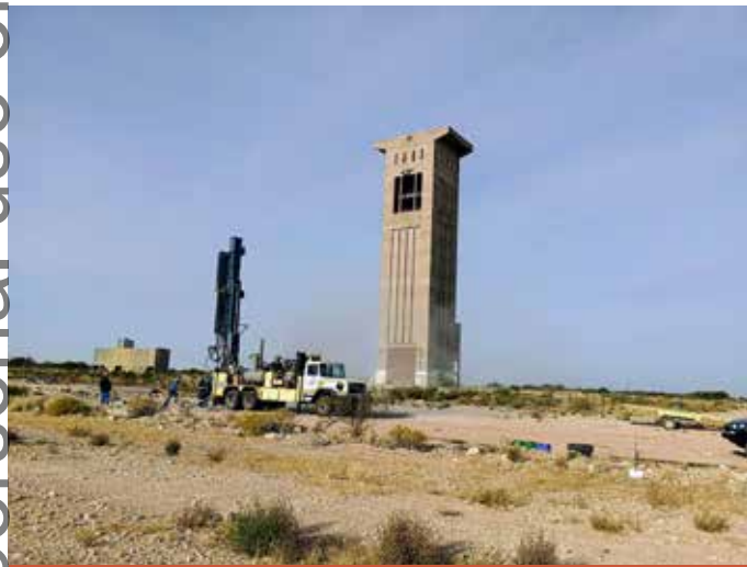
Figure 1: Drilling in progress for installation of rising main pump column from the 178 Level
