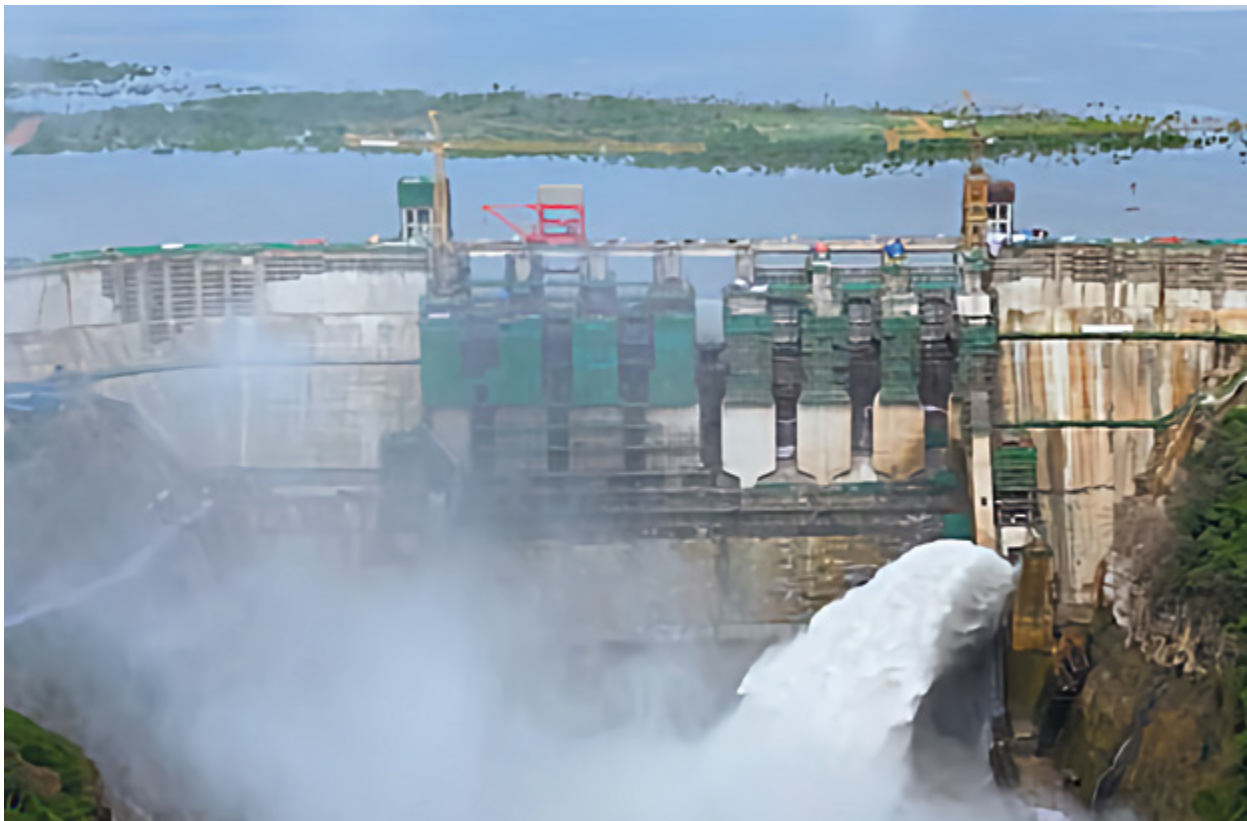
Photo 1 - The 2115MW Julius Nyerere Hydropower Project is expected to begin power generation soon
