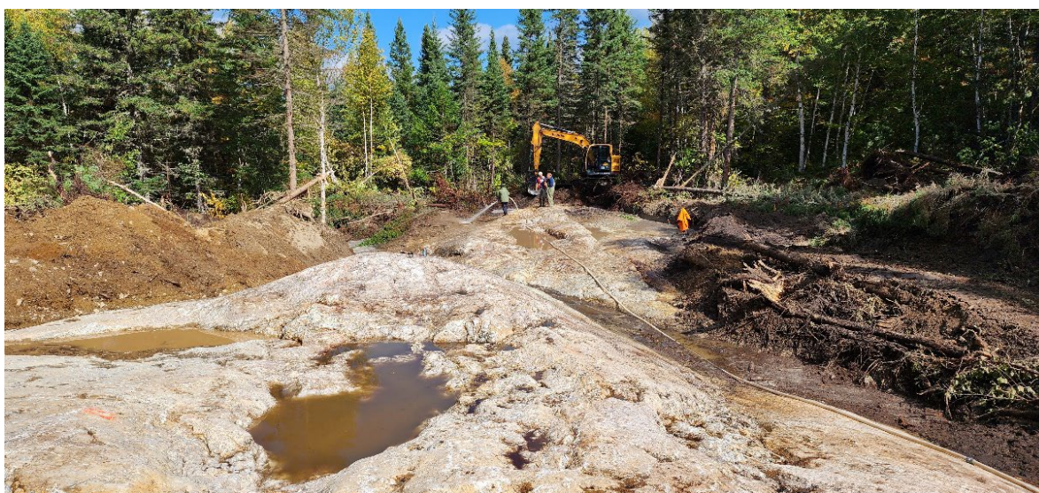
Figure 2 – Mechanical stripping underway at Nelson occurrence, Gorge Project
