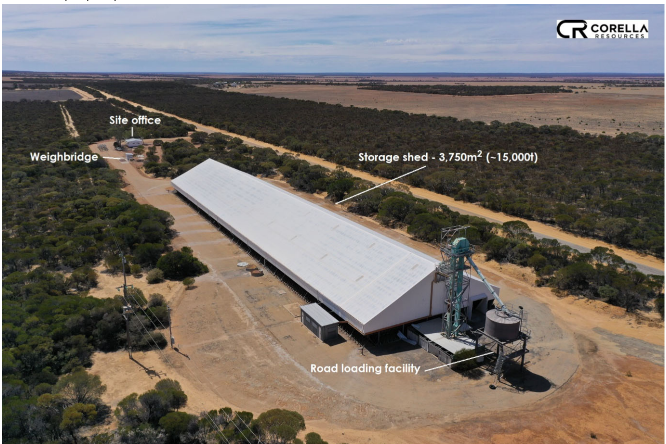
Figure 3: Tampu storage facility (view looking NNE)
