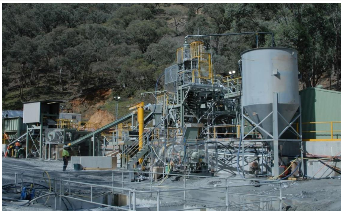
Figure 2 Hill End Gravity Gold plant
