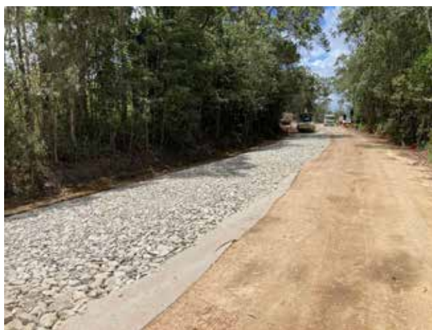
Euluma Creek Roadworks.
