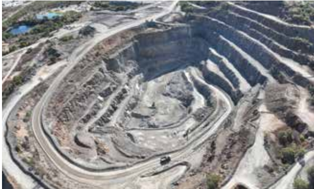
Commencement of open cut mining operations.
