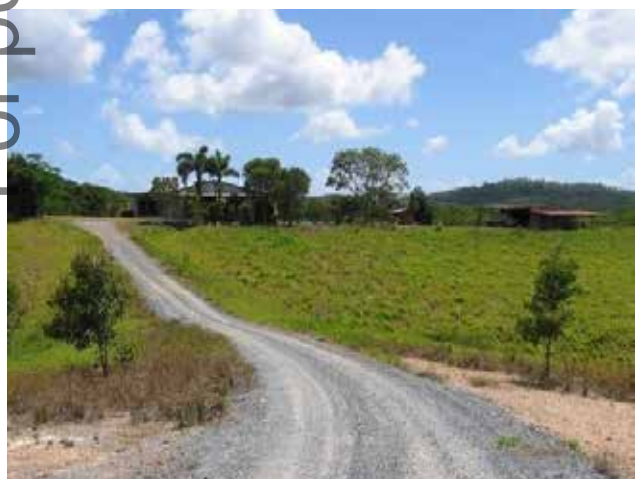
Julatten Road Rebuild.
