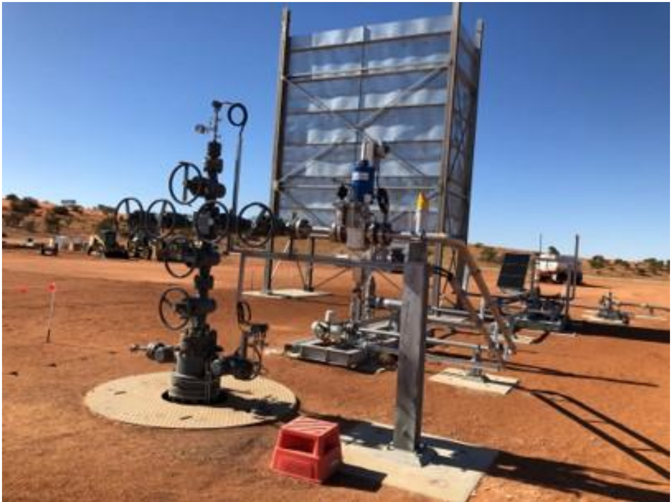
Vali-1 wellsite configuration
