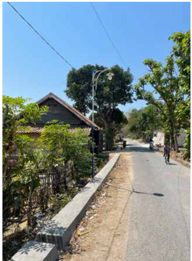
Sampang PSC: village external lighting installation
