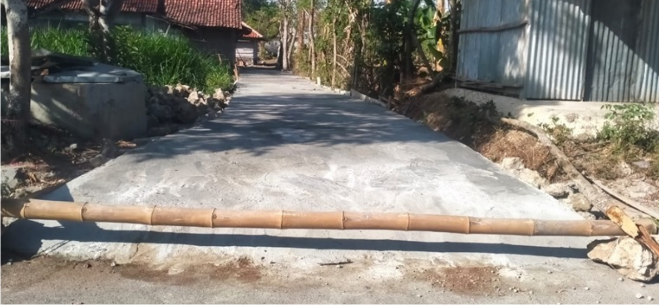
Sampang PSC: Road Construction in Banajar Talela village
