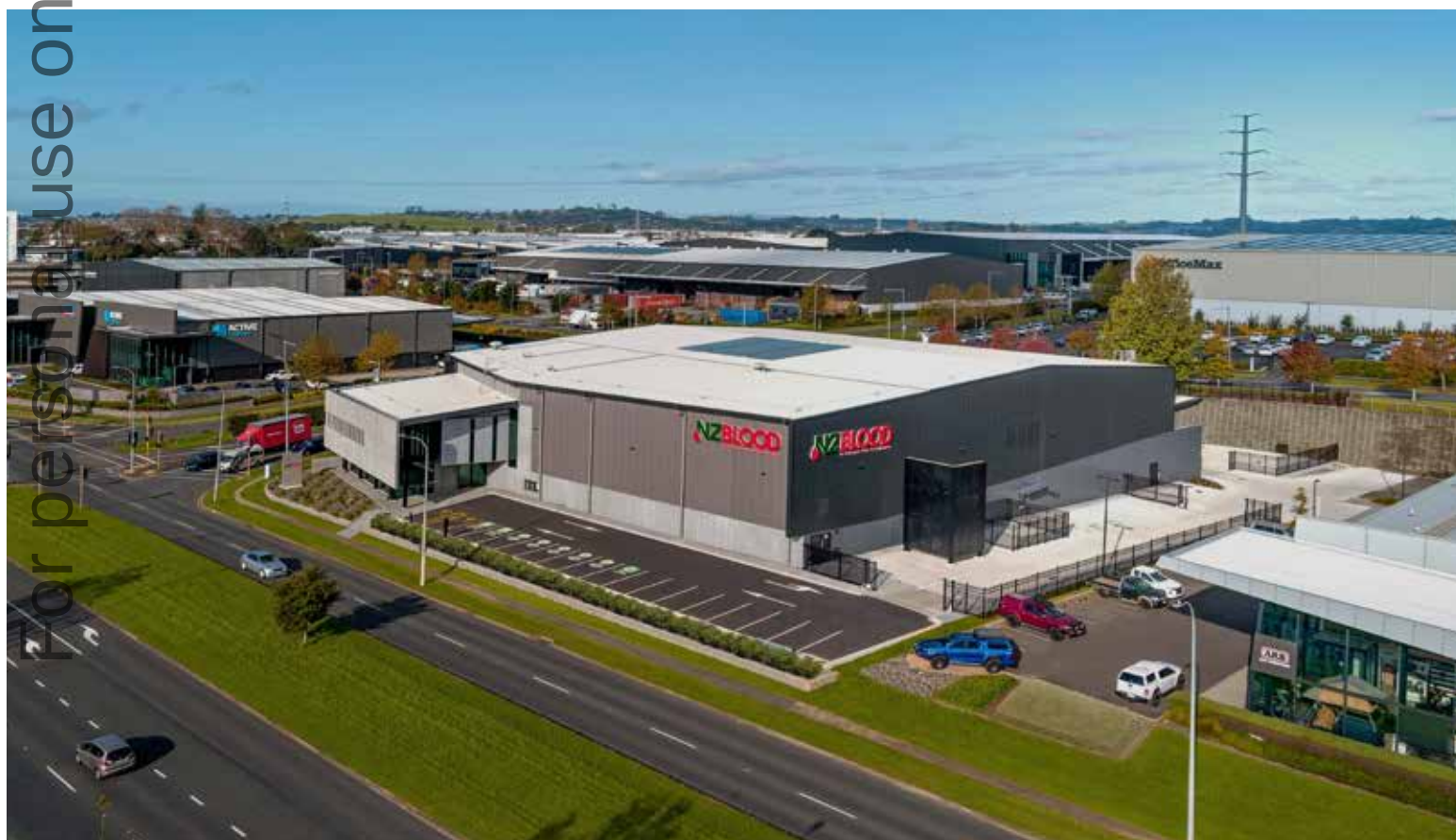
Highbrook Business Park, Auckland, New Zealand.
