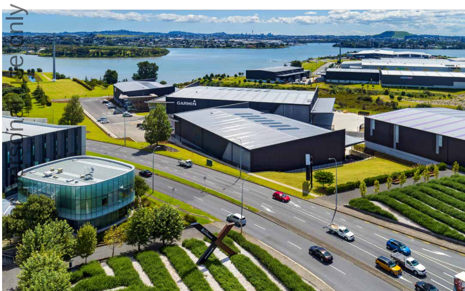
Highbrook Business Park, Auckland, New Zealand.
