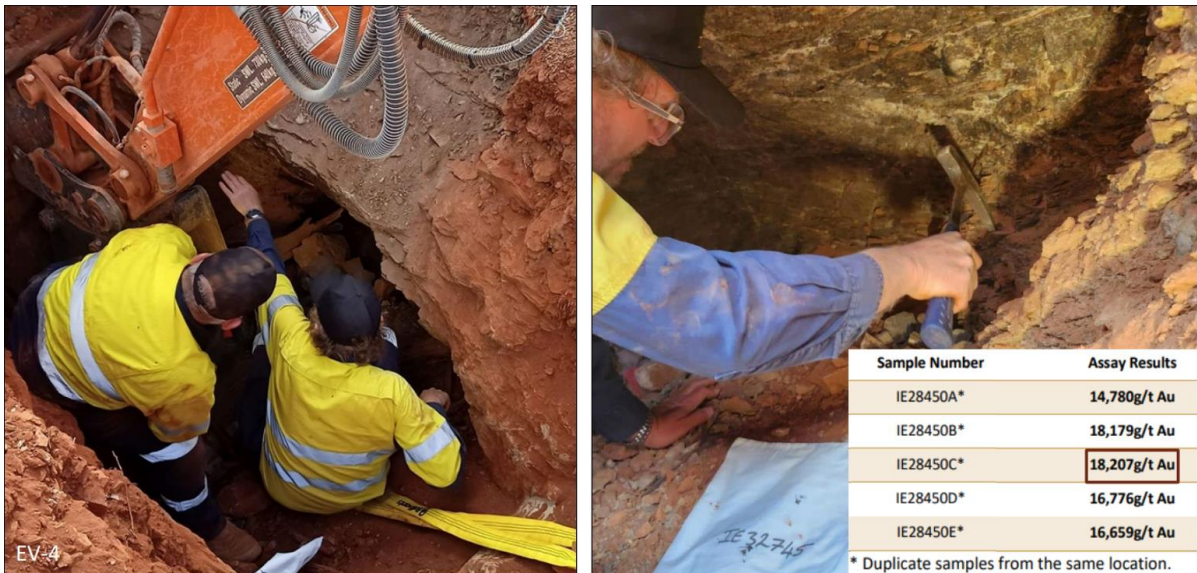
Figure 7: Inspecting the underground workings along strike from the Christmas Gift high-grade gold vein (from ASX release dated 16 June 2023).
