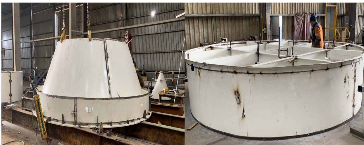
Workshop Fabrication of Spray Roaster Reactor Shell and Oxide Bin
