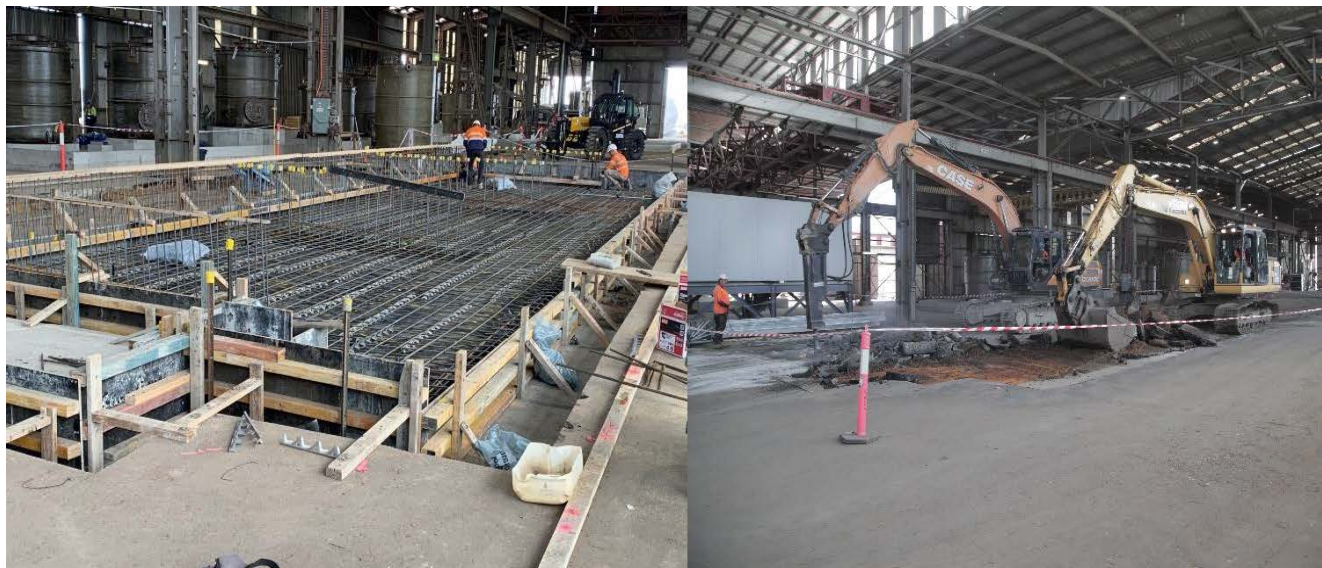
Figure: Filtration Area Formwork (left) and Filtration Area Excavation (right)
