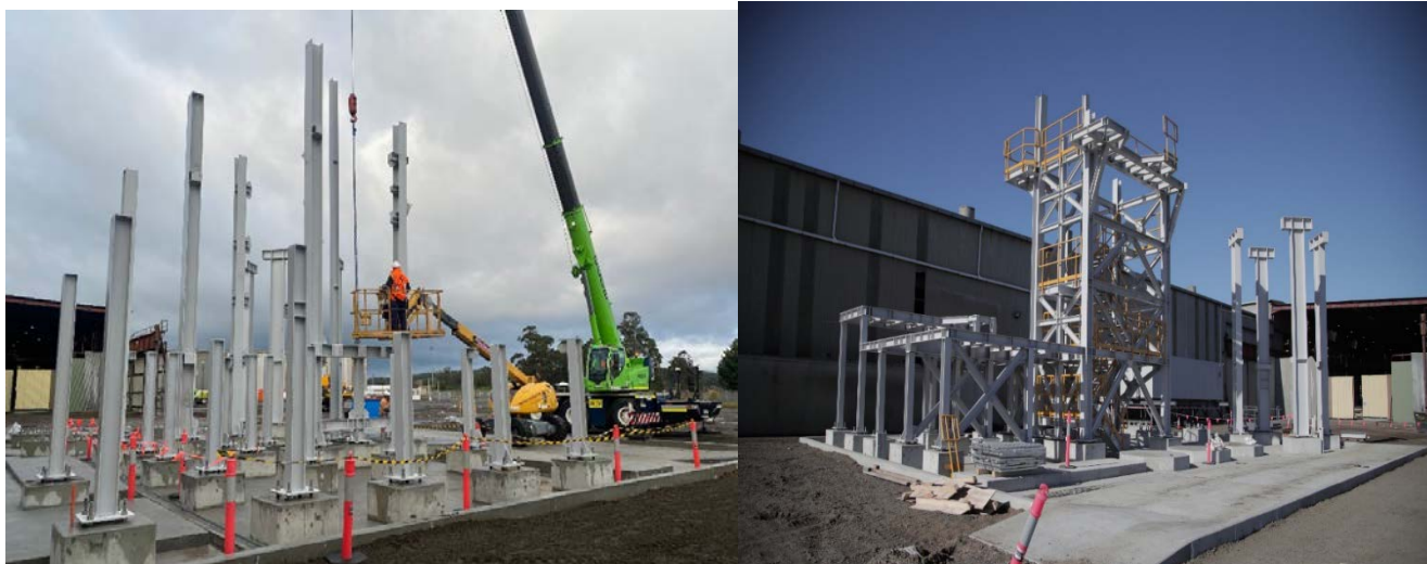
Spray Roaster Structural Steel Erection and Level 1 Erection
