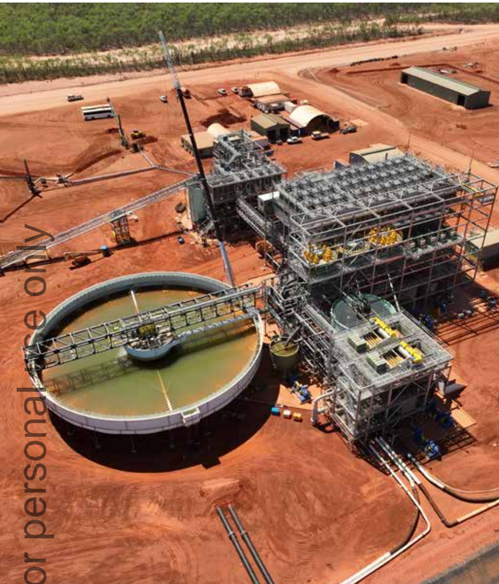
Figure 1: Construction in progress at the Thunderbird Mineral Sands Project
