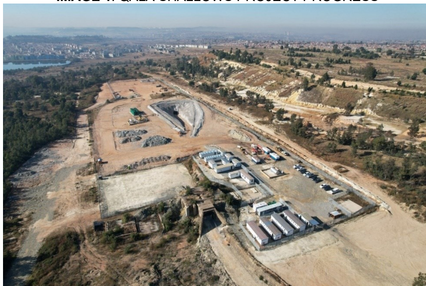
IMAGE 1: QALA SHALLOWS PROJECT PROGRESS
