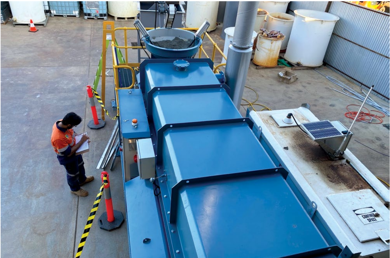
Figure 7 – Demonstration Plant. Commissioning of the kiln with concentrate
