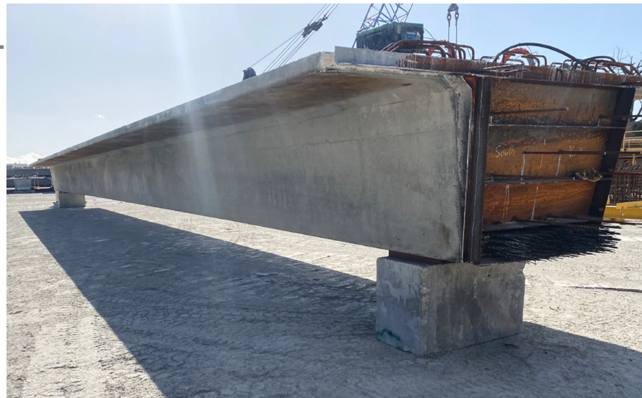
First beam cast in new multipurpose, high-capacity adjustable stressing bed – Bennett Brook Bridge
