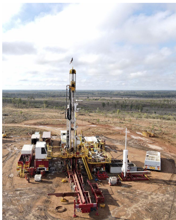
Figure 7 – Drilling Mahalo North 2 lateral well
