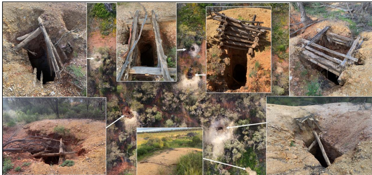
Figure 8: Mine shafts and workings at Creamy Hills gold mine (AGC ASX 3 March 2023).
