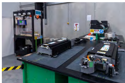
Infinitev battery testing station
