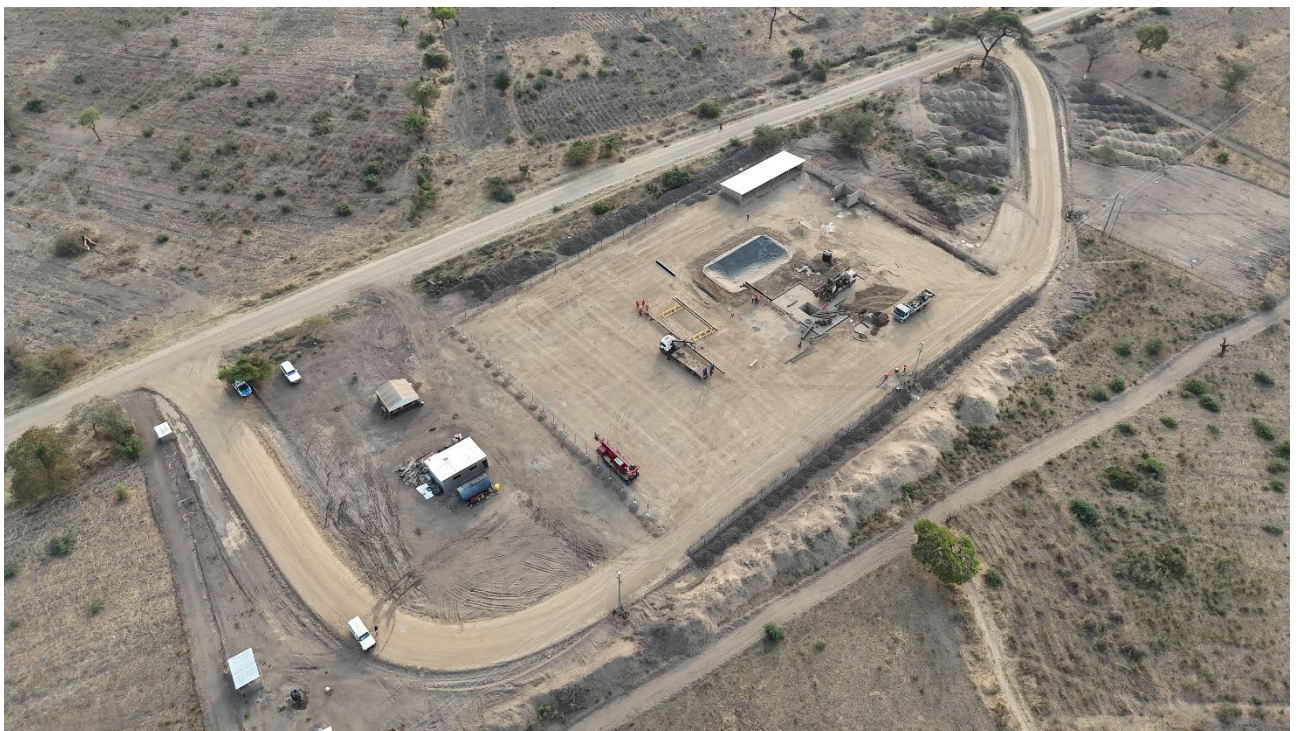
Figure 1. Mbelele-1 well site complete and ready for drilling to start in late September.
