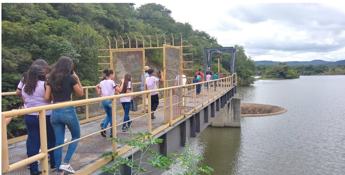
Figure 13: Students visit the Curralinho Dam spillway
