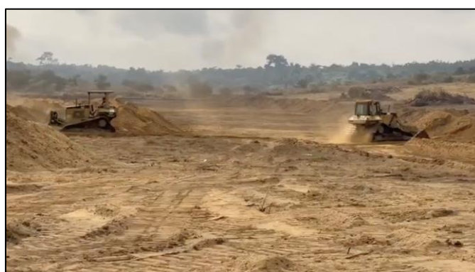
Figure 1 - Earthworks underway at Subantando, site of the Cabinda Phosphate Fertilizer Factory.
