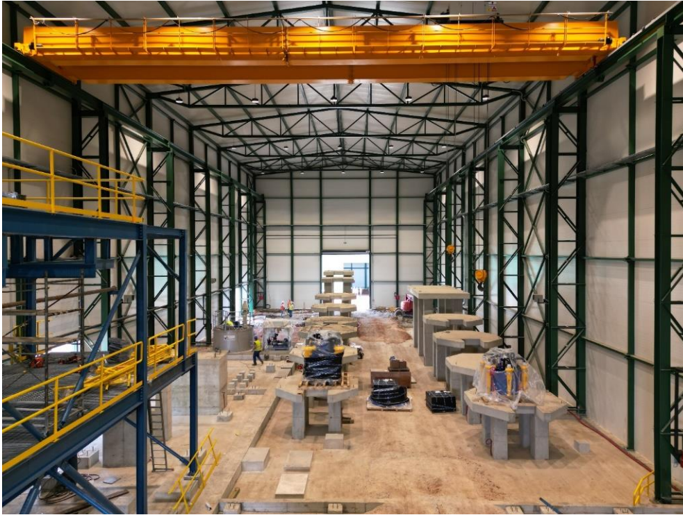
Figure 6: Flotation building, July 2023
