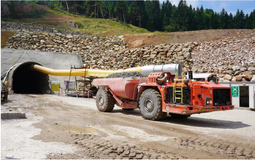
Figure 3: Lower Decline Portal
