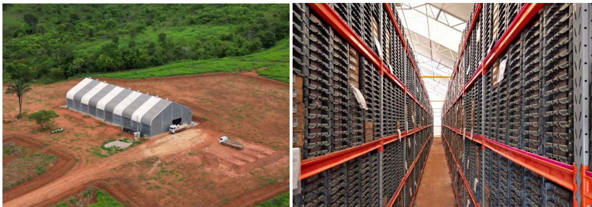
Figure 2 – New Core Shed at Jaguar
