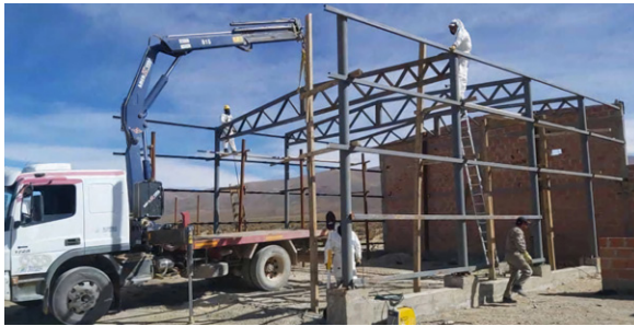
Hydro crane assistance for building of workshop – Olaroz Chico
