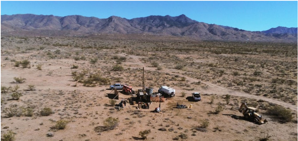
Figure 3: Diamond drilling at the Tintic prospect at the Kingman Gold Project, Arizona – November 2022.
