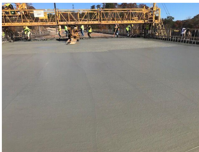
Figure 13. Little River bridge trial- showing freshly installed concrete in 2019
