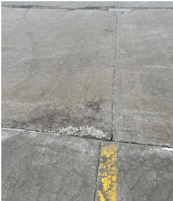
Figure 3. Section of worn concrete
