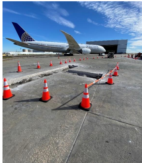
Figure 4. Concrete slabs being replaced
