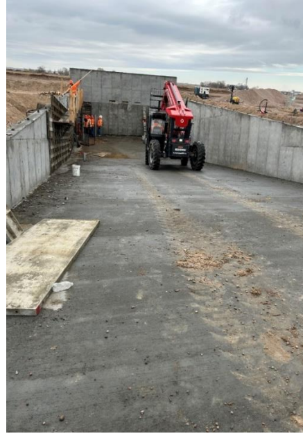
Figure 10. Longs Peak Dairy-fluid retention basin with walls.
