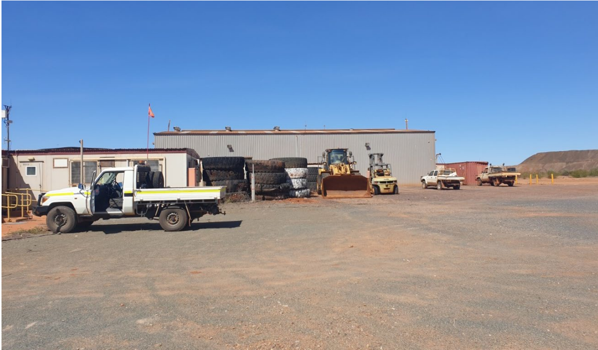
Figure 25: Whim Creek Project existing main office workshop
