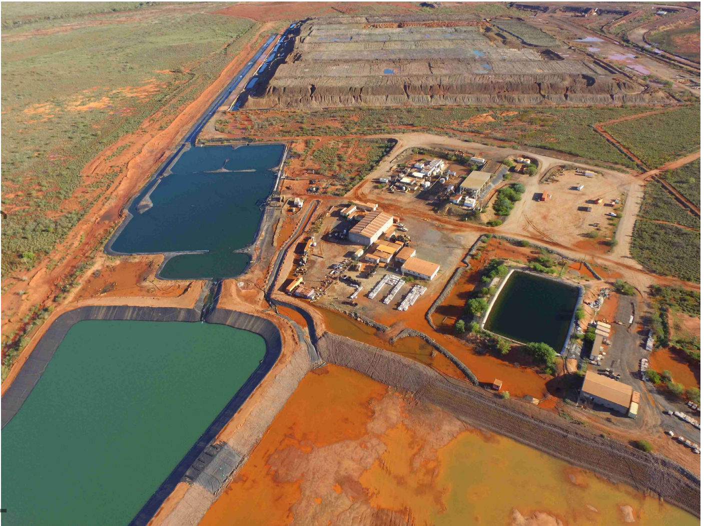
Figure 1: Whim Creek Heap Leach and Associated Infrastructure
