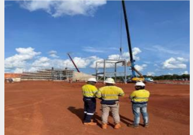
Structure for primary crusher discharge
