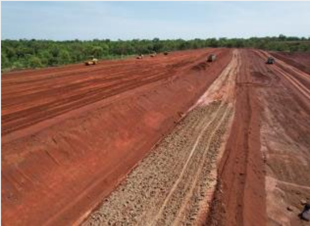
TSF embankment construction
