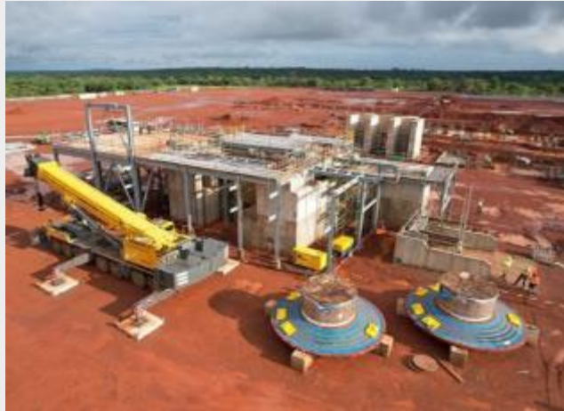
450 t crane in position for mill installation
