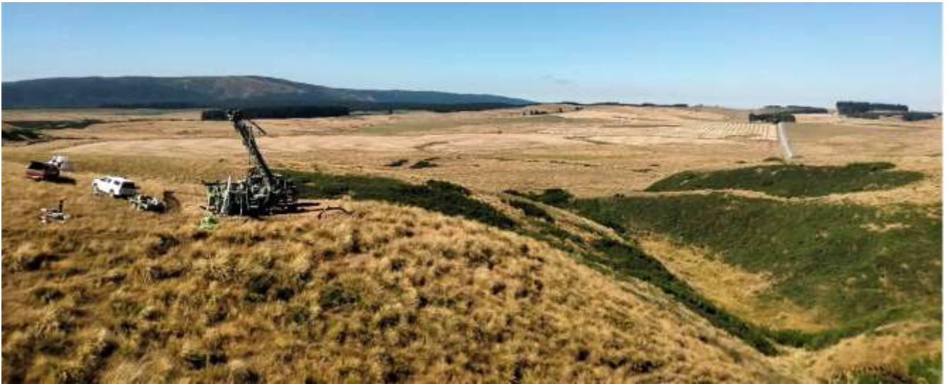
Figure 10: OPQ drilling rig looking south
