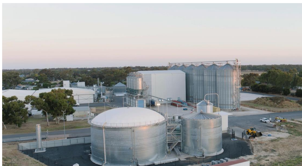
Image 3: Blue Lake Milling bioenergy facility
