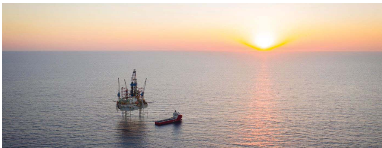
Figure 2: Image of Noble's Tom Prosser rig on site during the Dorado Appraisal campaign.
