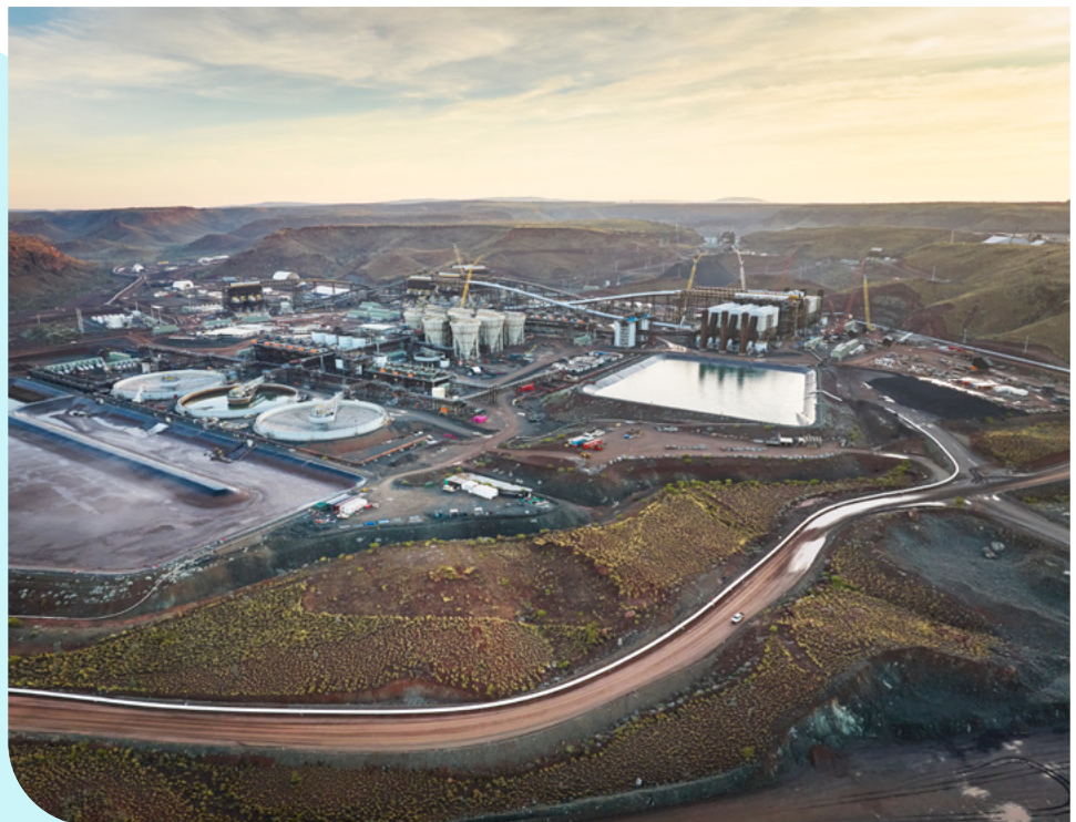
Iron Bridge Project
