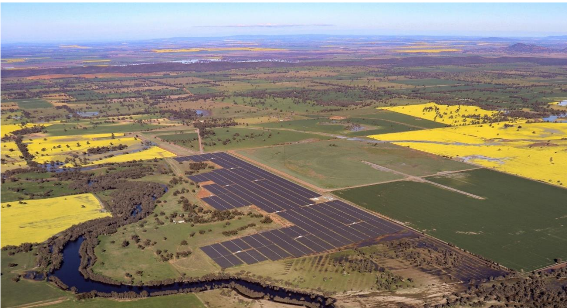
Above: 50MW Jemalong Solar Farm, Central NSW
