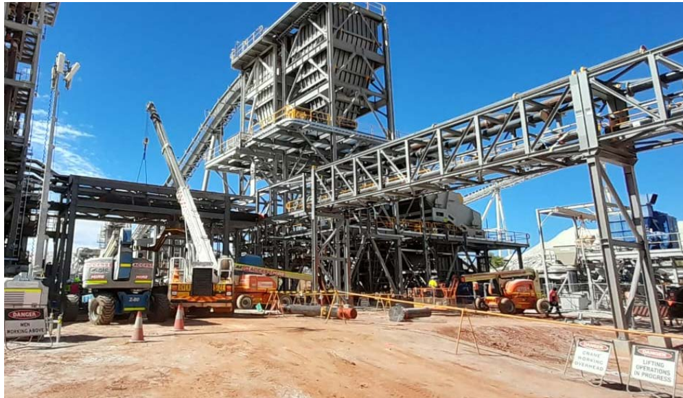
Image: P680 Project - Primary rejection infrastructure construction underway
