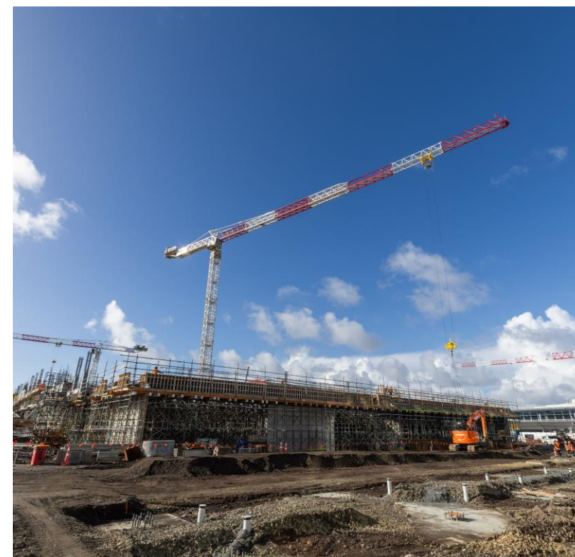
Construction of the Transport Hub
