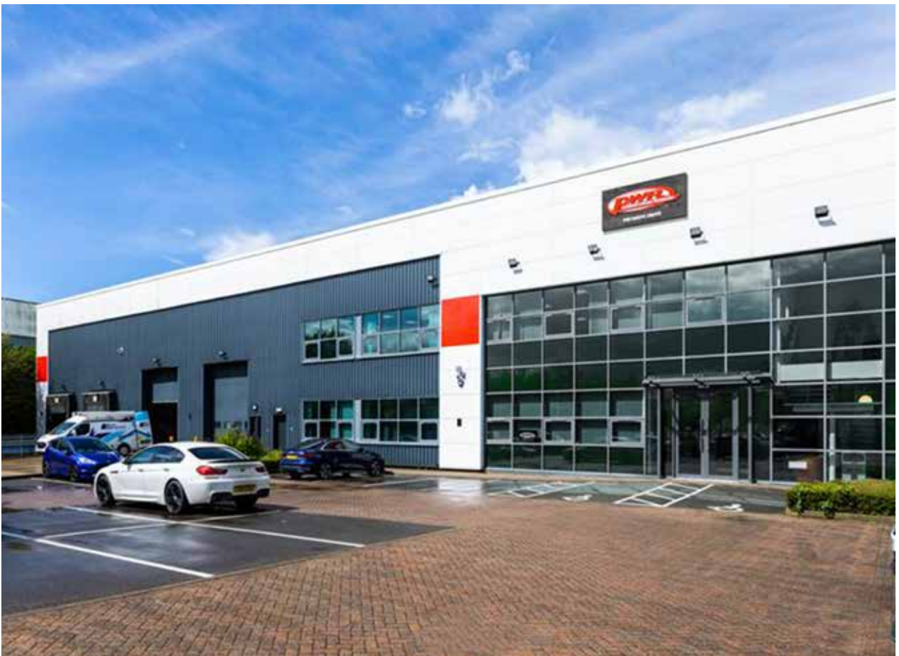
PWR Europe's new manufacturing facility located in Rugby, United Kingdom
