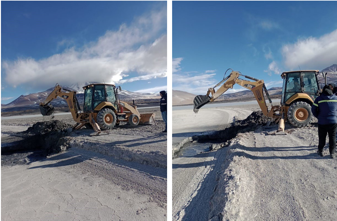
Figure 2 Preparing drilling fluid supply for SJDD01, San Jorge Project
