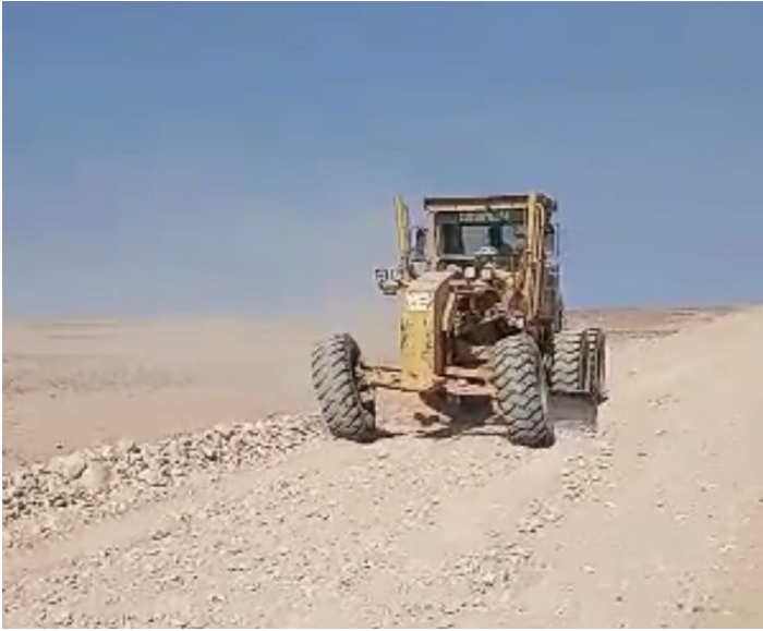
Figure 3: Work on access track improvements in-progress.
