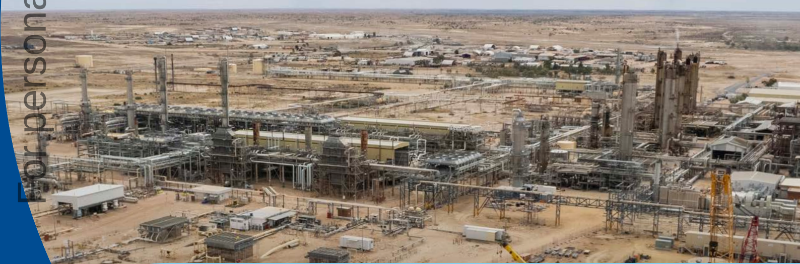
→ Moomba CCS construction
