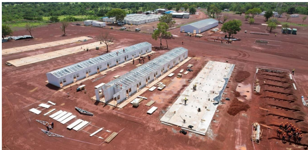
Image 9 - Construction of permanent accommodation facility, with pioneer facility in back.
