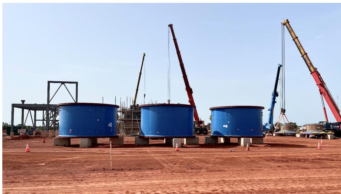
Image 8 - Ball mill components received on site.
