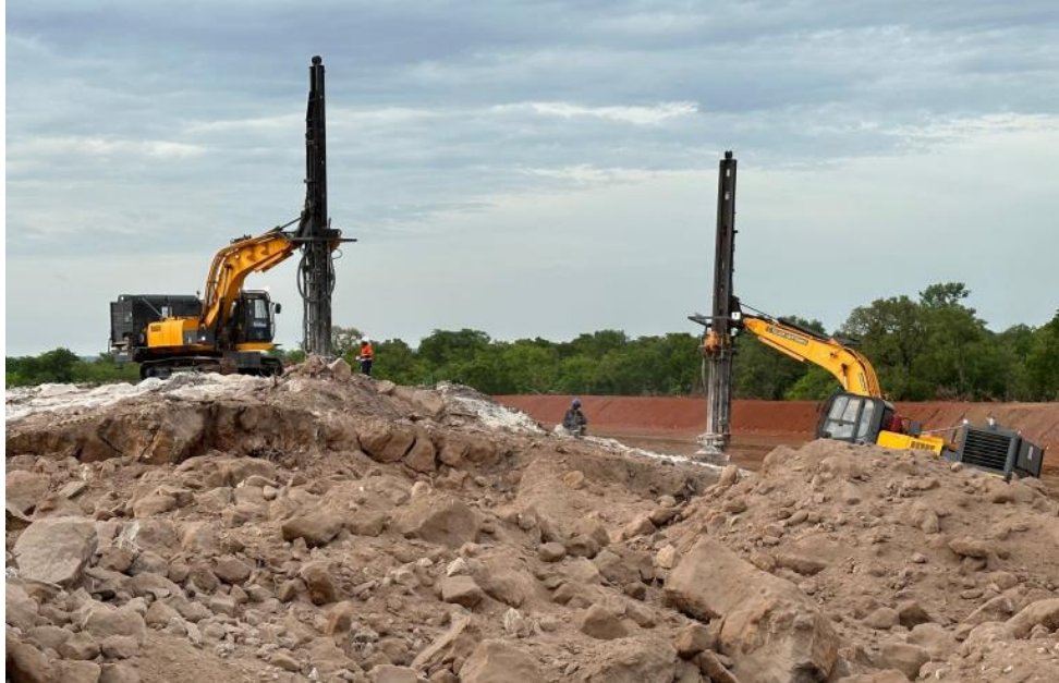
Image 6 - Mining contractor mobilised initial fleet.
