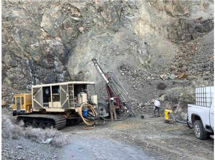
Figure 4 Drill rig on hole IM14A.
