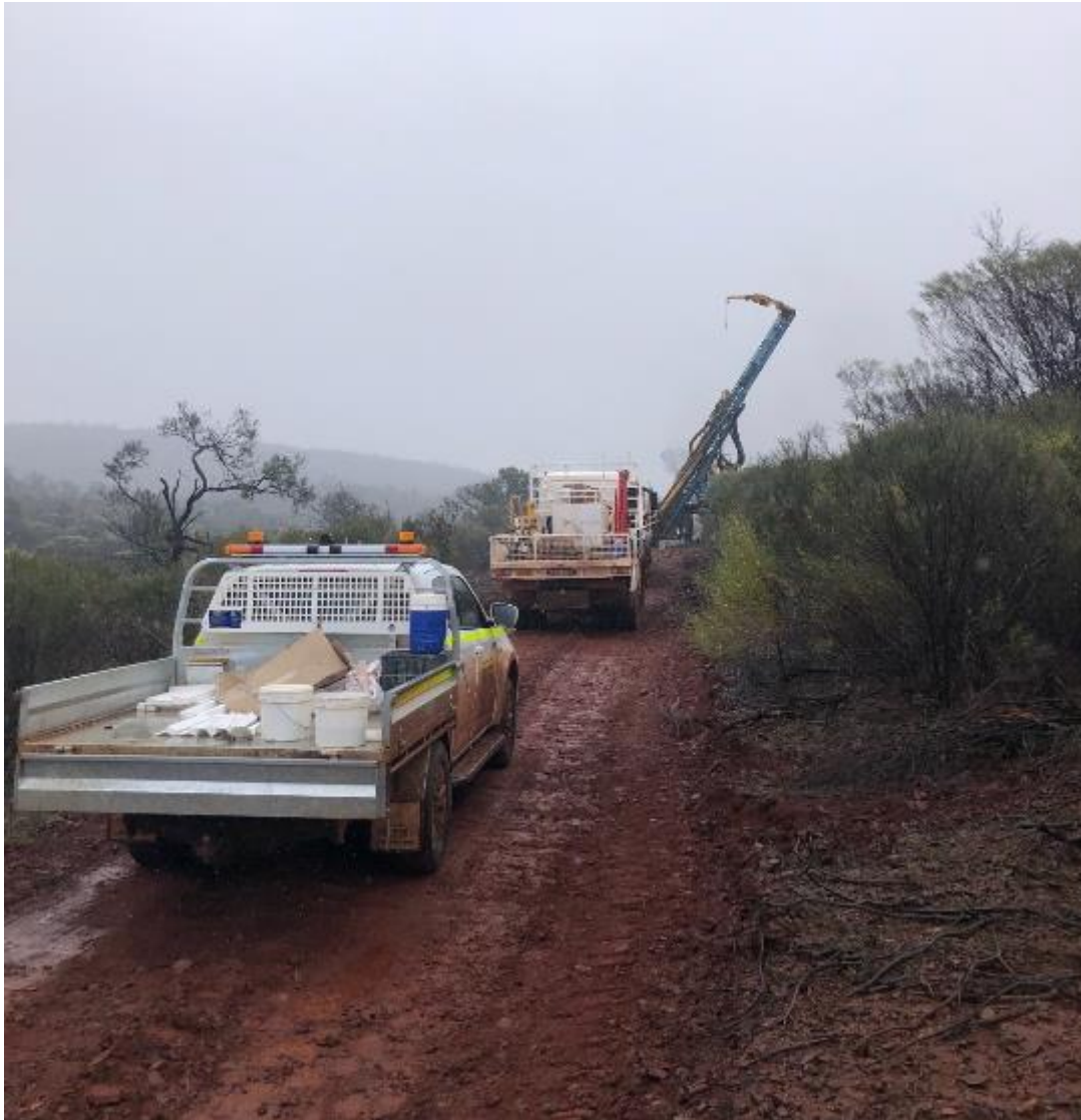
Picture 2. Smokebush RC Drilling at the Monza IP target.
